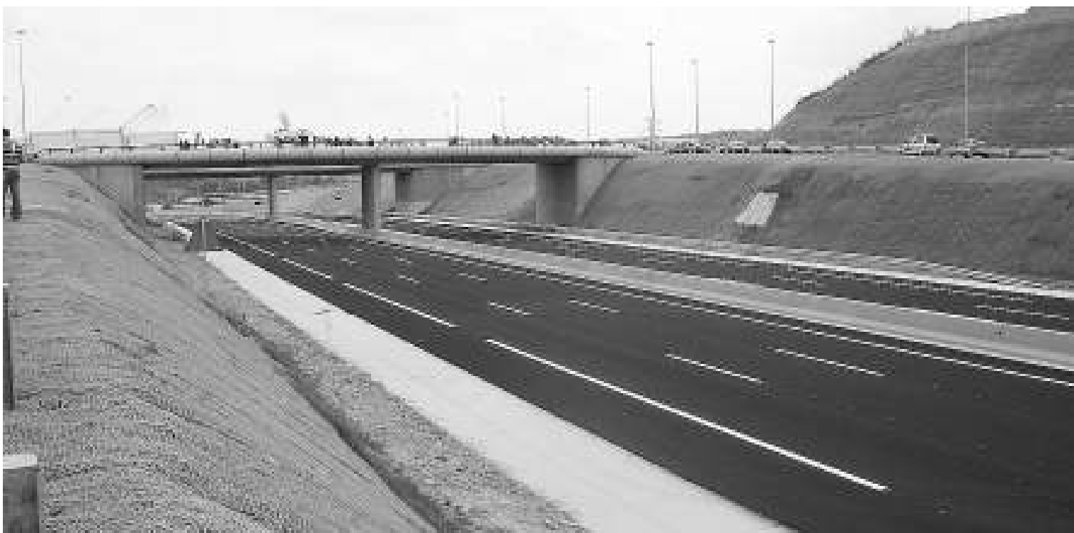
The new ten-kilometre A-2 dual carriageway section between Panadella and Santa María del Camí is expected to receive a daily volume of 26,000 vehicles / SEGRE
