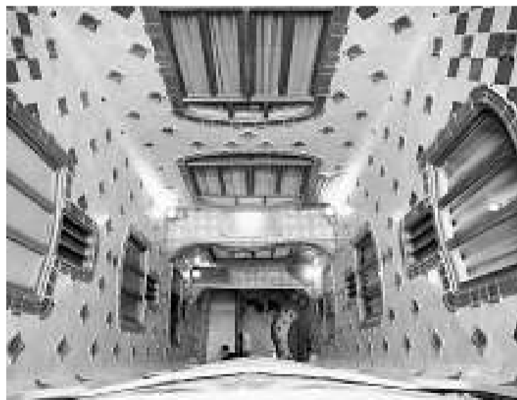
Panoramic view of central lift shaft. / GABRIEL MASSANA
