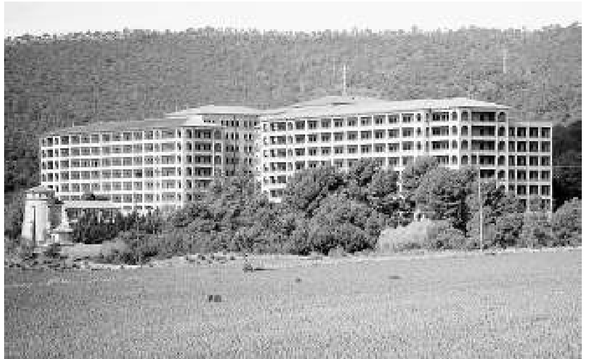
The new media complex, including the Filmoteca archives, will be housed in this former hospital in Terrassa / OSCARESPINOSA
