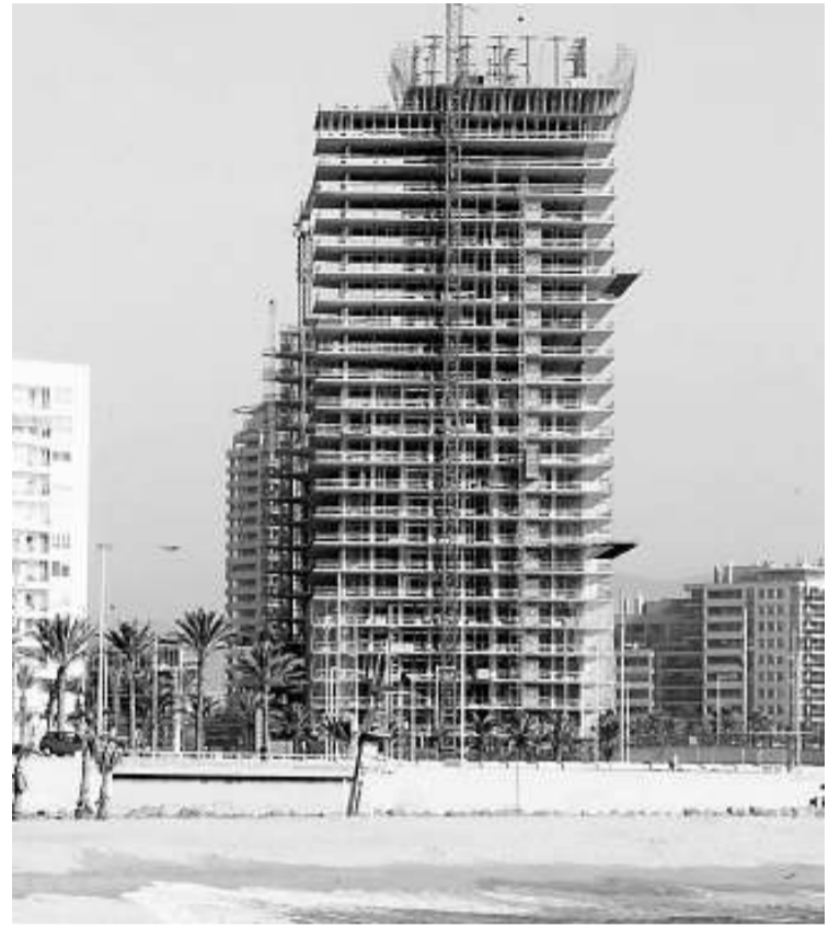
The city is stepping away from high rises towards private homes
